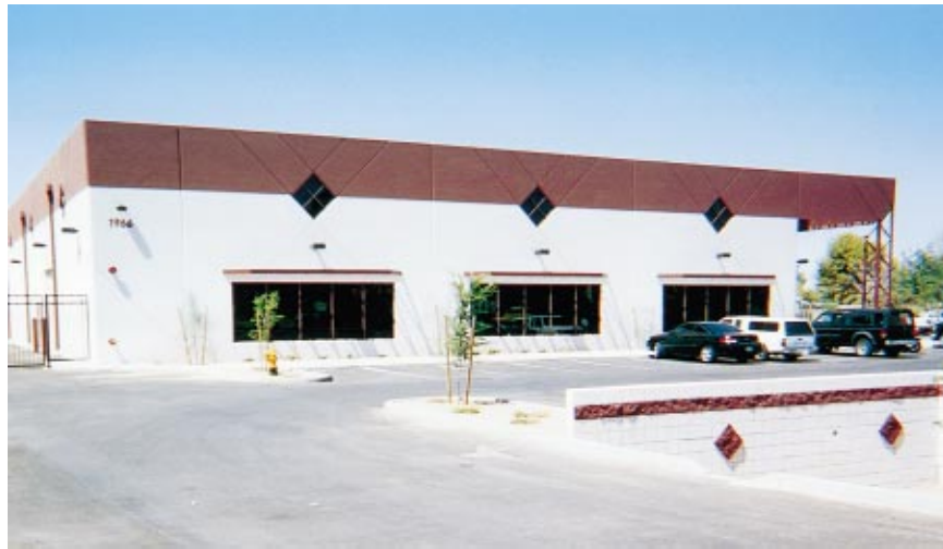
Fig. 13. (Color) Finished building
