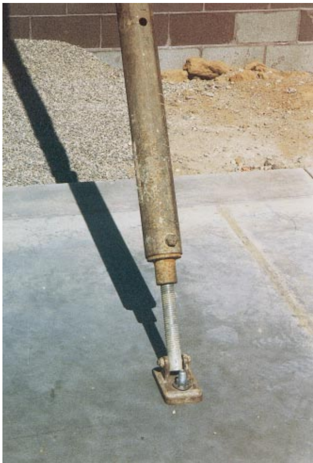
Fig. 10. (Color) Extendable end of a Burke brace
