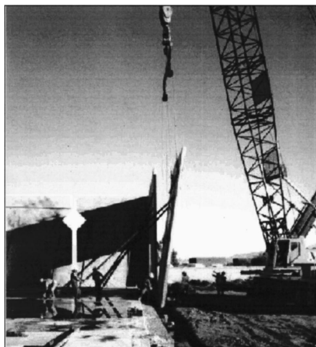
Fig. 12. Mobile lattice boom crane (300 t) erecting panels
