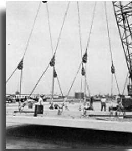
Lifting A Panel
