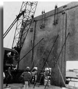
Bracing A Panel
