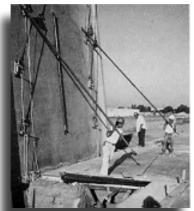
Bracing A Panel
