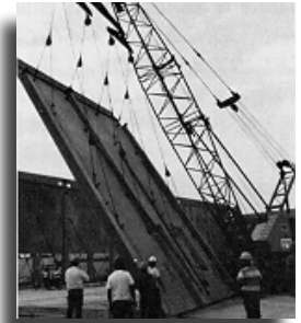
Lifting A Panel
