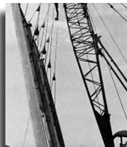
Placing A Panel
